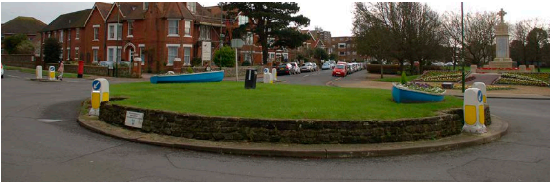
Large inaccessible, raised roundabout blocks views, hiding approaching vehicles.
