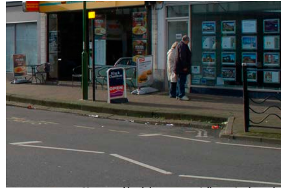
Unexpected level changes potentially causing hazards to the pedestrian and reducing movement opportunities.
