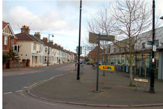
Nondescript and under performing space formed at junction between New Road and Pier Road.
