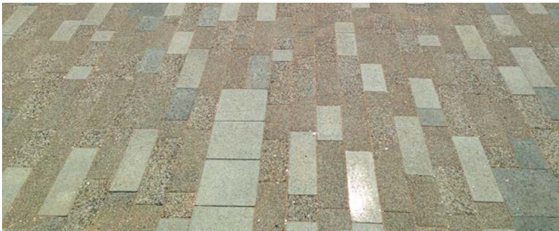
Randomised laying patterns providing a characteristic mixture of texture and a unique appearance whilst being structurally capable as performing it's desired functions
