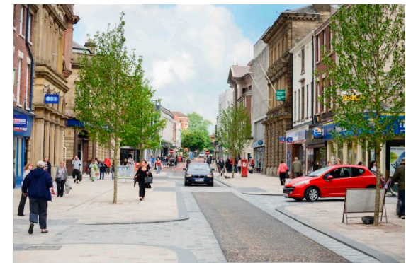
Fishergate, Preston; Shallow kerb to highlight pedestrian 'safe-zone'.
