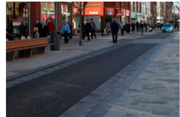
Fishergate, Preston; Wide channels providing the illusion of a narrower carriageway. Shallow upstand kerb to define pedestrian only zone.
