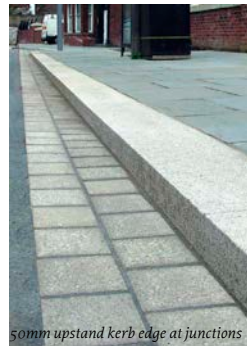
somm upstand kerb edge at junctions
