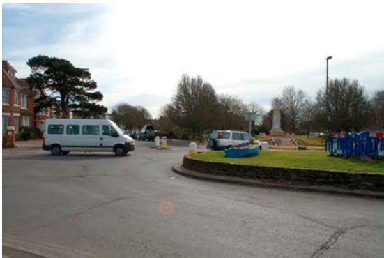
Desire lines blocked and movement restricted.
