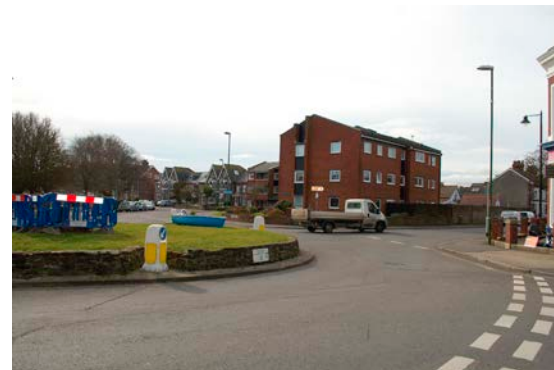
Odd shaped roundabout provides complication for vehicle users and pedestrians alike.
